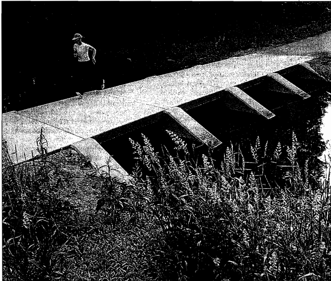
A pedestrian uses the bridge to cross the stream under the bike path that runs near the Great Miami River and the bridge at east Ohio 41. Due to consistent flooding, the bridge will be reconstructed. Staff photo by Jim Witmer
