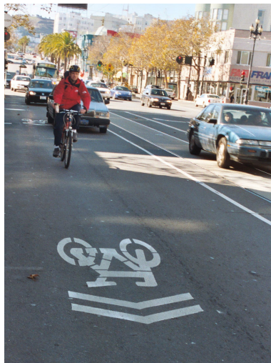
Alta conducted a shared-lane pavement markings study for the City of San Francisco as part of the city's bicycle master plan.
