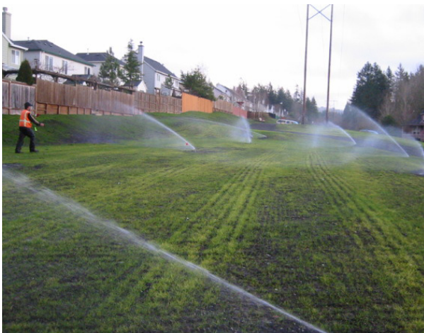
The successful test of a 24-zone irrigation system at Kaiser Woods Park, Beaverton, Oregon. The park program included planting, irrigation, trail design, and site furnishings.
