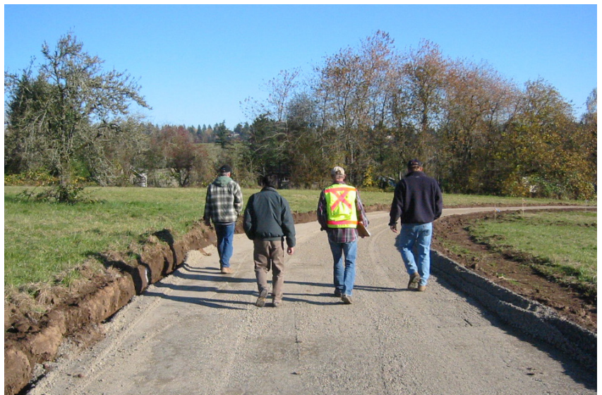
Principal George Hudson joins the contractor, client, and City Engineer on a weekly site inspection of the Stafford Basin Pathway in Lake Oswego, Oregon. Regular site visits during construction will keep a project on schedule and allow early identification and quick resolution of issues.
