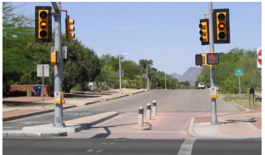
Signalization techniques, such as this “toucan” signal, allow cyclists to safely and comfortably cross intersections.
