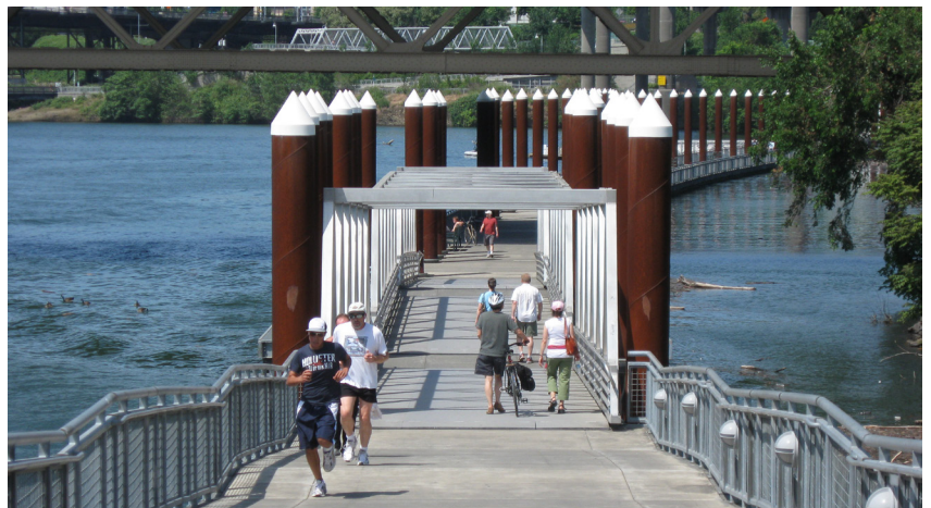
Alta Principal George Hudson managed the design and construction of the Eastbank Esplanade in Portland, Oregon. It includes a floating trail section on the Willamette River, ramps to the Burnside Bridge, and a connection to the Steel Bridge bicycle/pedestrian cantilevered path and the Willamette River Water Trail.
